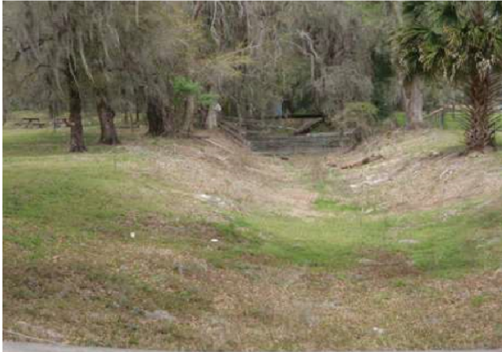
Figure 2: Dade City Canal in Florida is a man-made, mostly dry conveyance for flood control. Dade City Canal is not currently a water of the United States but would likely be deemed a “tributary” under the Rule. Fla. Stormwater Ass’n Comments 10, ID-7965 (JA__).
