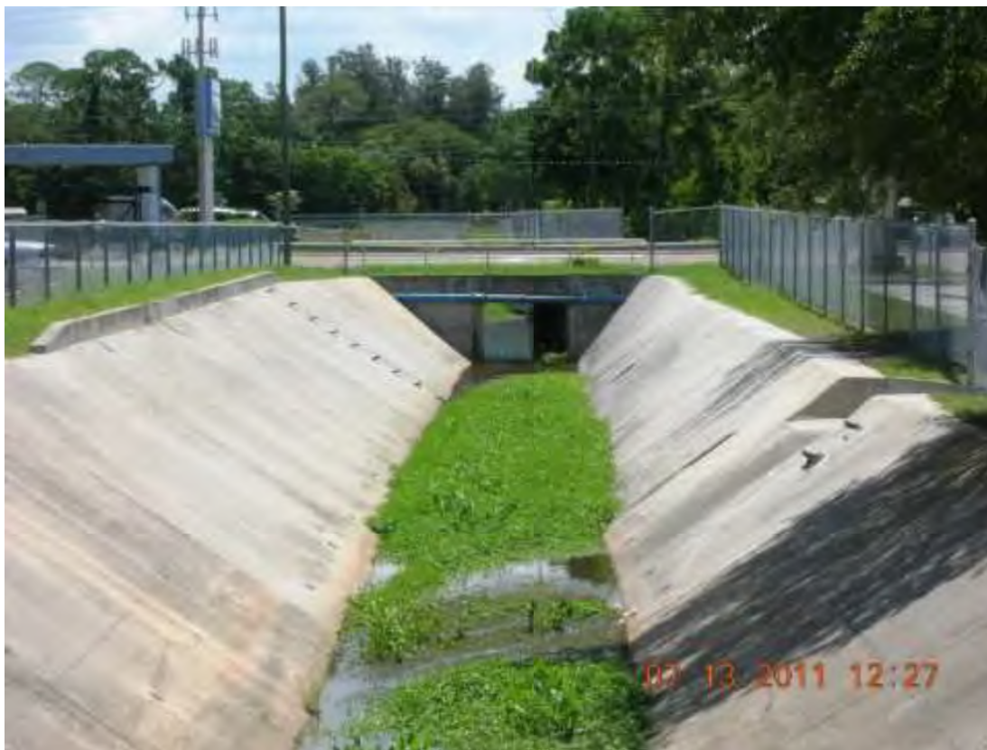
Figure 6: Ditch #5 in Pinellas County, Florida, is a manmade stormwater conveyance that discharges through a wetland into a navigable creek. It is already regulated as a point source. Under the Rule, it will be additionally regulated as a “water of the United States.” Fla. Stormwater Ass’n Comments 13 (JA__).
